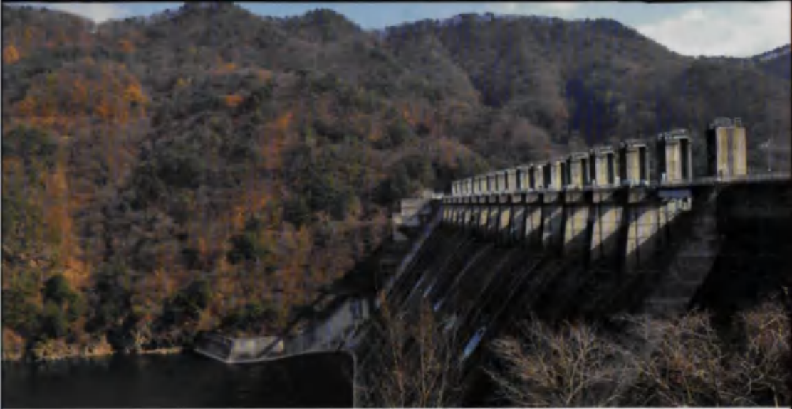
Hwacheon Dam, built by the Japanese between 1939 and 1944
