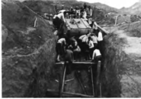
Excavation work at the Yin Ruins
