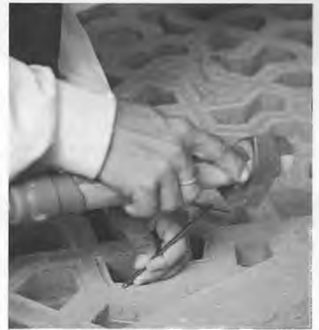
A stonemason doing restoration work
