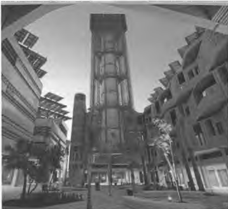
Centre Courtyard and wind tower at the Masdar Institute
