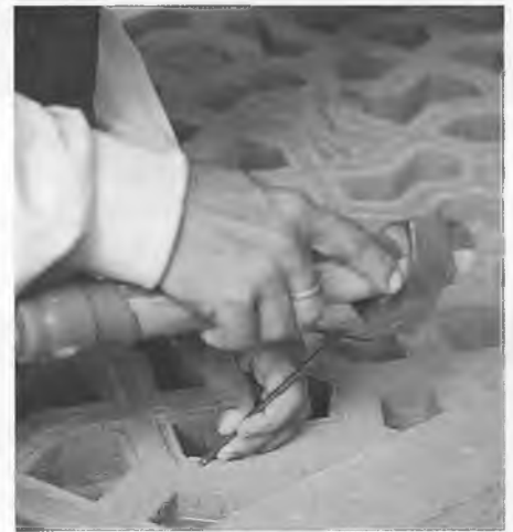
A stonemason doing restoration work
