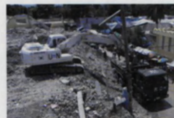
The Danbi Unit performing restoration work [June 2010]
