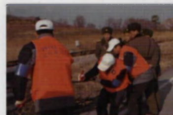
Construction to Upgrade inter-Korean Military Communications Lines
