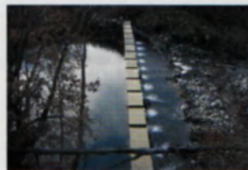
Regulating Reservoir Dam
