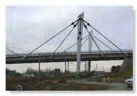
The four cable forces are all concurrent at point O on this bridge tower, Consequently they produce no resultant moment there, only a resultant force  $F_R$ . Note that the designers have positioned the cables so that  $F_R$  is directed along the bridge tower directly to the support, so that it does not cause any bending of the tower.
