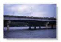
To save on material and thereby produce an efficient design, these beams, also called girders, have been tapered, since the internal moment in the beam will be larger at the supports, or piers, than at the center of the span.
