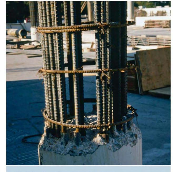
These reinforcing rods will be encased in concrete in order to create a building column. The internal loadings developed within the material resist the external loading that is to be placed upon the column.
