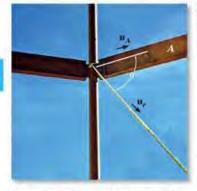
The angle  $\theta$  between the rope and the connecting beam can be determined by formulating unit vectors along the beam and rope and then using the dot product  $\mathbf{u}_h \cdot \mathbf{u}_e = (1)(1)\cos\theta$ .
