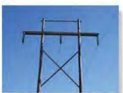
In order to design the beam used to support these power lines, it is important to first draw the shear and moment diagrams for the beam.
