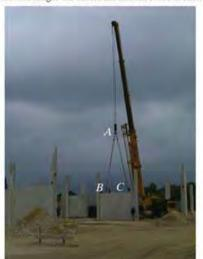
P3-2. The truss is hoisted using cable ABC that passes through a very small pulley at B. If the truss is placed in a tipped position, show that it will always return to the horizontal position to maintain equilibrium.
