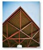
Typical roof-supporting space truss. Notice the use of ball-andsocket joints for the connections
