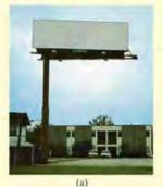
The uniform sign shown in Fig. 7-8a has a mass of 650 kg and is supported on the fixed column. Design codes indicate that the expected maximum uniform wind loading that will occur in the area where it is located is 900 Pa. Determine the internal loadings at A.
