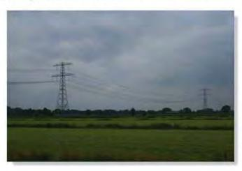
Electrical transmission towers must be designed to support the weights of the suspended power lines. The weight and length of the cables can be determined since they each form a catenary curve.
