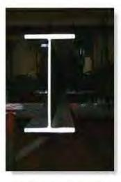
In order to predict the strength and deflection of this beam, it is necessary to calculate the moment of inertia of the beam's cross-sectional area.
