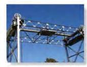
The use of metal gusset plates in the construction of these Warren trusses is clearly evident.
