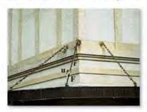
The force  $\mathbf{F}$  acting along the chain can be represented as a Cartesian vector by establishing x, y, z axes and first forming a position vector  $\mathbf{r}$  along the length of the chain. Then the corresponding unit vector  $\mathbf{u} = \mathbf{r}/r$  that defines the direction of both the chain and the force can be determined. Finally, the magnitude of the force is combined with its direction,  $\mathbf{F} = F\mathbf{u}$ .
