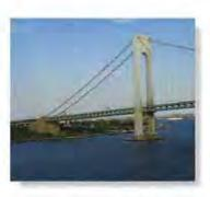
The cables of the suspension bridge exert very large forces on the tower and the foundation block which have to be accounted for in their design.
