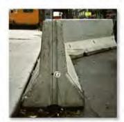
In order to determine the force required to tip over this concrete barrier it is first necessary to determine the location of its center of gravity G. Due to symmetry, G will lie on the vertical axis of symmetry.
