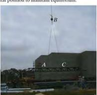
P3-3. The device DB is used to pull on the chain ABC so as to hold a door closed on the bin. If the angle between AB and the horizontal segment BC is  $30^{\circ}$ , determine the angle between DB and the horizontal for equilibrium.
