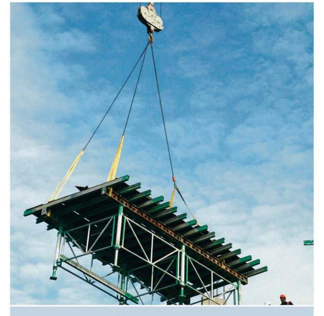
Whenever cables are used for hoisting loads, they must be selected so that they do not fail when they are placed at their points of attachment. In this chapter, we will show how to calculate cable loadings for such cases.
