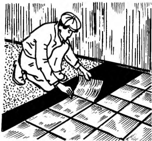
109-rasm. Plitkalarini sovuq mastikada yopishtirish.
