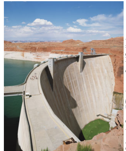
Glen Canyon Dam at Lake Powell, Arizona
