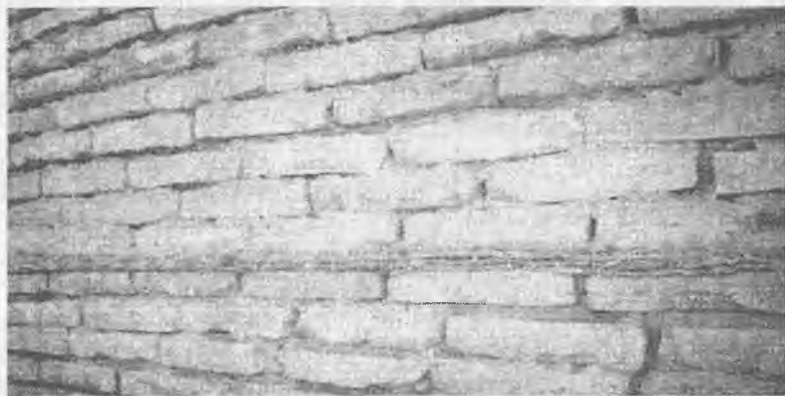
63-rasm. Binolar poydevorida qamish qatlamidan foydalanish.
