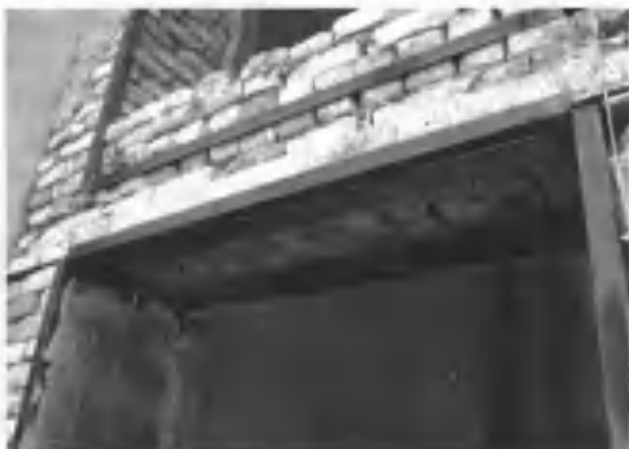
2.11-rasm. Proyoamlarni o'rash (obramlenie) yo'li bilan bino prostenkalarini kuchaytirish.
