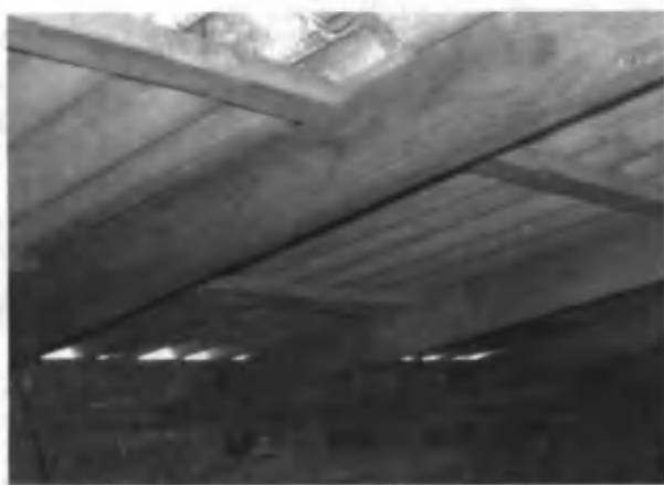
1.58-rasm. Chordoqli tomda to'sinning tagsinchiga, panjara (obreshyotka)ning to'singa o'rnatilishi.
