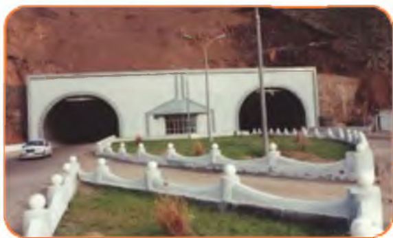
69-rasm. Qamchiq dovonidagi tunnel.
