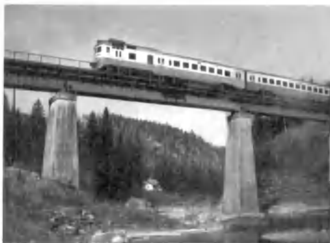
5.22-rasm. Viaduk ustidan poyezd o'tishi
