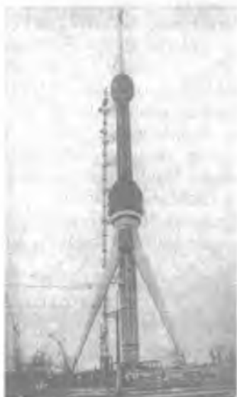
19.7-rasm. Toshkent shahridagi 350m.li teleminora.
