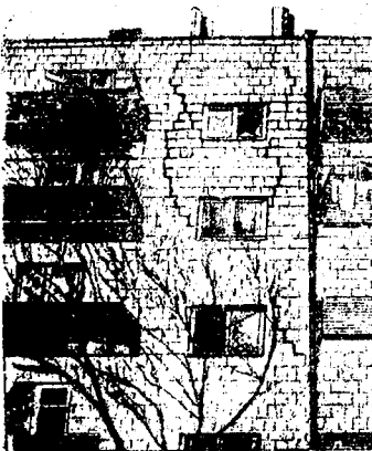
14.2-rasm. Zaminning o'ta cho'kishi natijasida yorilgan bino.
