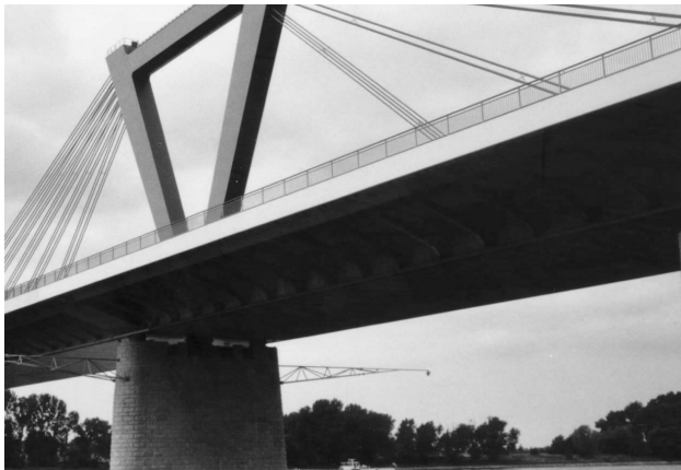
22-rasm. Dansig, Polsha: shosseli ko'prik, erituvchanligi oz miqdorli Icosit-Proxicolor® va Icosit® EG 4 materiallari bilan ta'mirlangan
