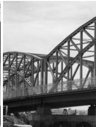
22-rasm. Dansig, Polsha: shosseli ko'prik, erituvchanligi oz miqdorli Icosit-Proxicolor® va Icosit® EG 4 materiallari bilan ta'mirlangan
